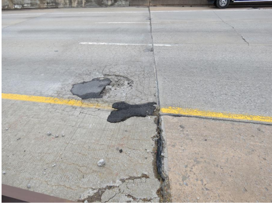
WEARING SURFACE "A" END W/ PATCHES
