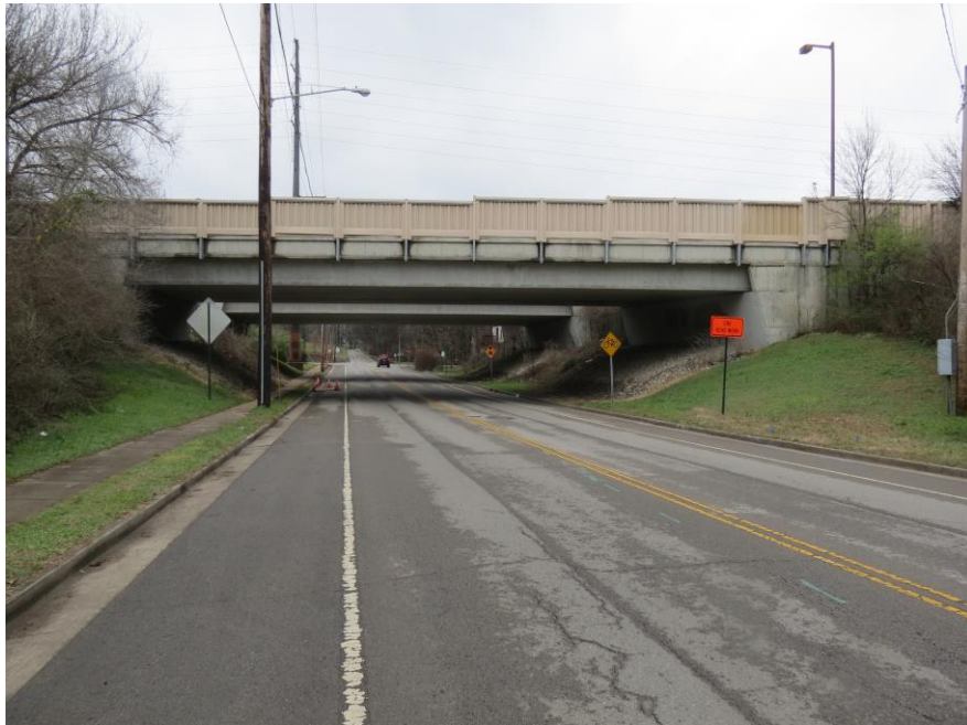
CLEARANCE VIEW RT. SIDE
