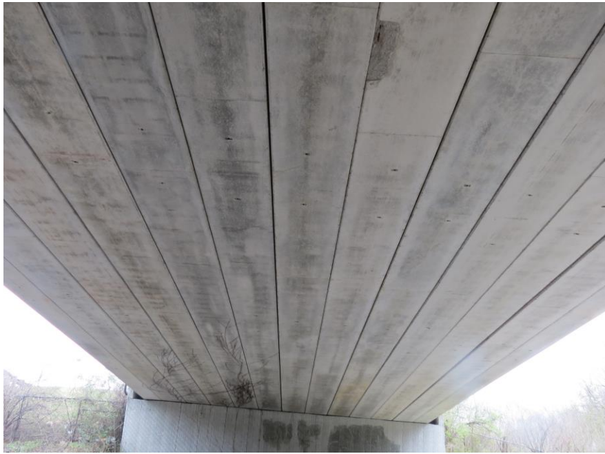
UNDERSIDE VIEW H.B.B.
